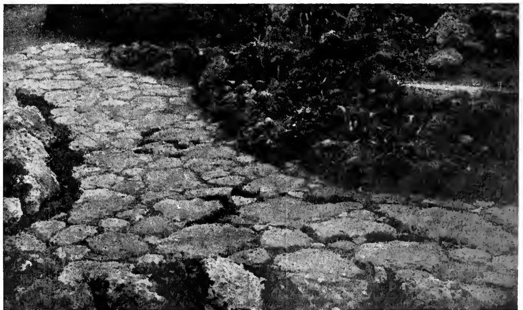
THE PATHWAY COMPLETED AND PARTIALLY FURNISHED WITH LOW-GROWING ALPINES.
